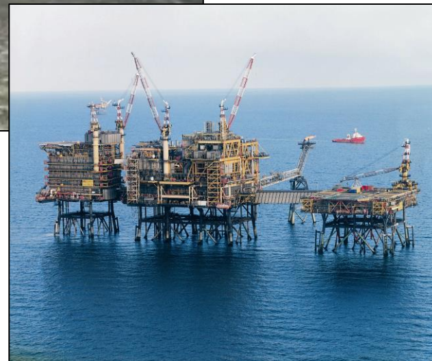
The Morecambe Gas Platform
